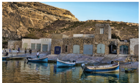
Quaternary deposits form the mound behind the boathouses at the Inland Sea
